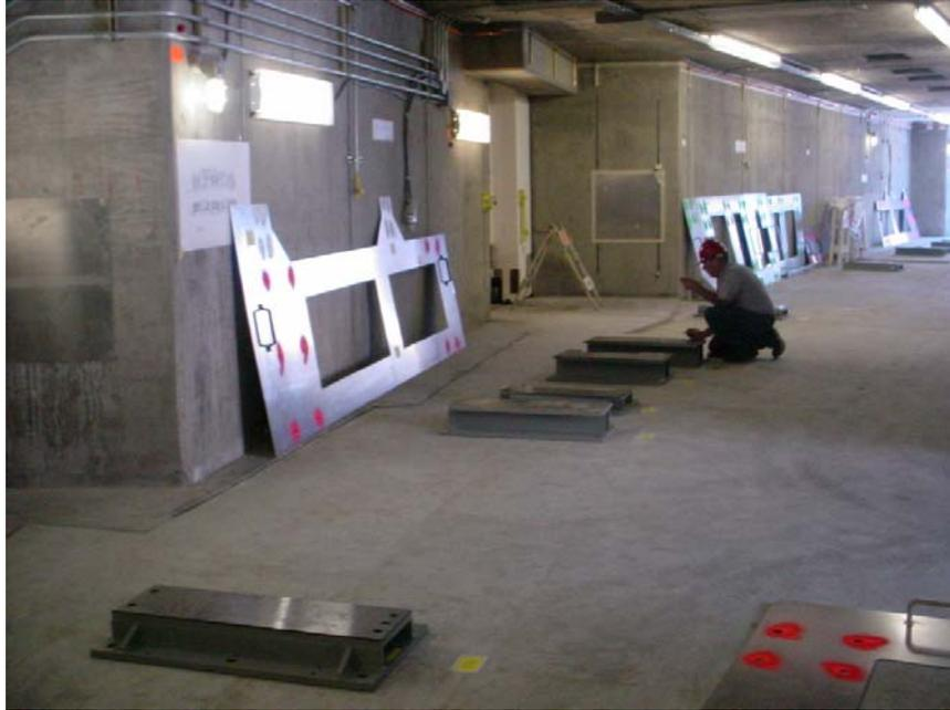
Raft support plates being placed onto marked holes- note hole templates in background
