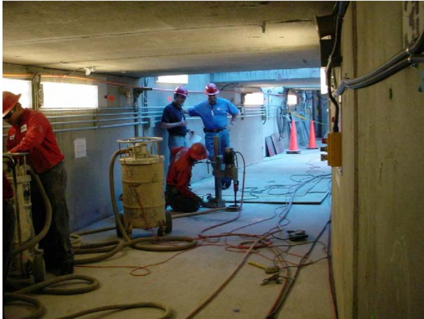
Core drilling of Raft & Straight section mounting holes
