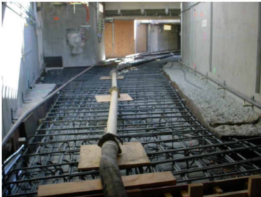
Quadrant 2 with rebar installed and ready to be poured
