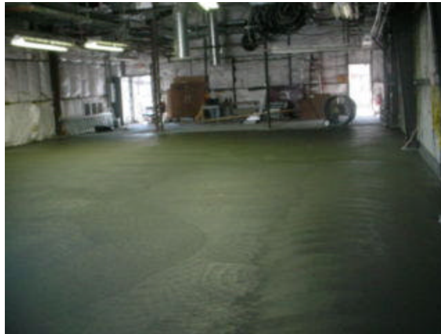
B118 concrete floor
