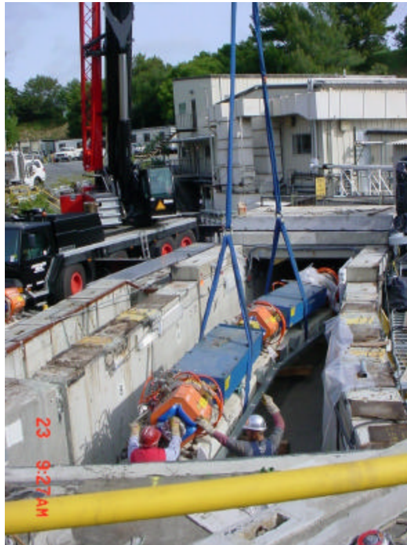
SPEAR2 Raft – removal from tunnel
