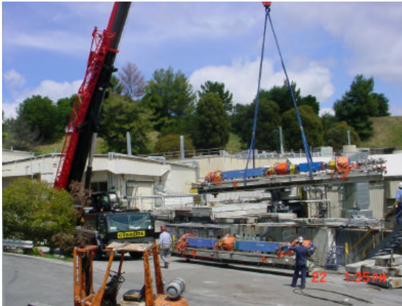
SPEAR 2 girders being removed from the ring housing
