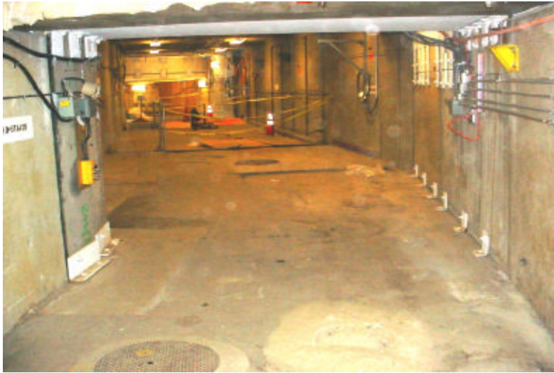
SPEAR tunnel near the end of April
