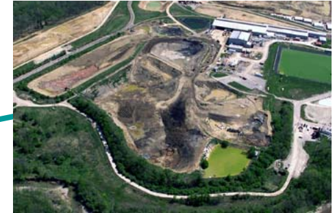
Waste Pits Fernald, OH
