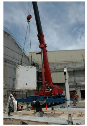
Phase one of the FFTB deconstruction (de-energizing energy sources and removal of key components) was completed on schedule on May. Phase two is now underway (removal of all accelerator components and supports, cabling and cable trays and concrete enclosure blocks). Phase two (see picture on right) is scheduled to be completed in late July.
