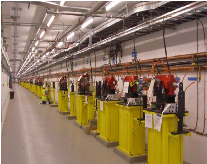
Beam Transport Hall
