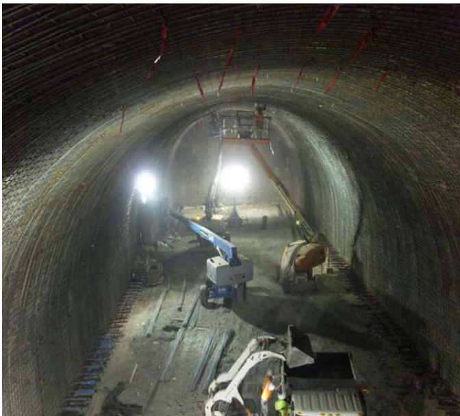
FEH final liner installation of rebar
