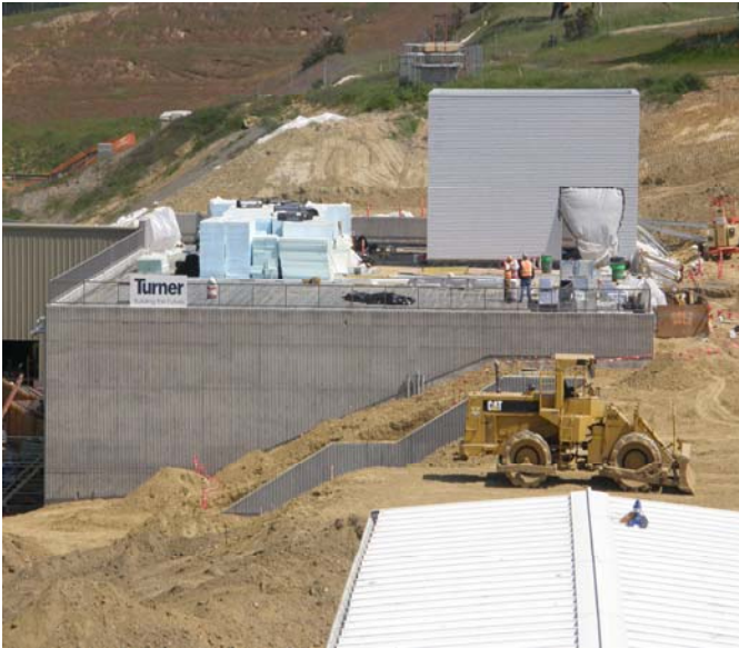
NEH with final grading
