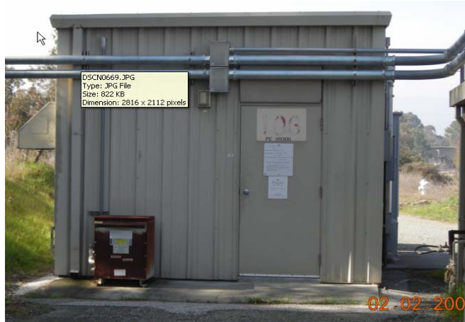
EXTERIOR VIEW OF BUILDING
