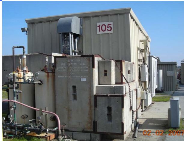
EXTERIOR VIEW OF EXISTING BUILDING
