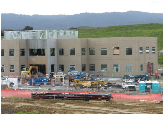
B901 exterior window installation
