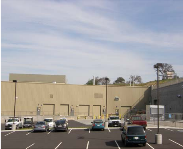
Central Utility Plant
