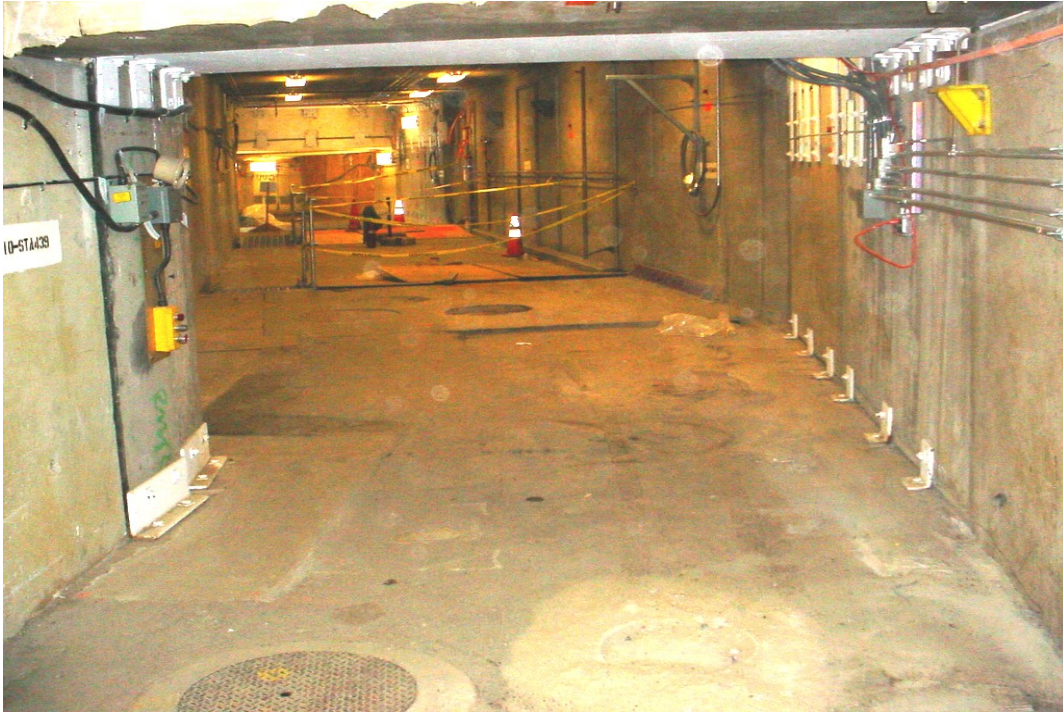
Figure 13 - SPEAR tunnel near the end of April
