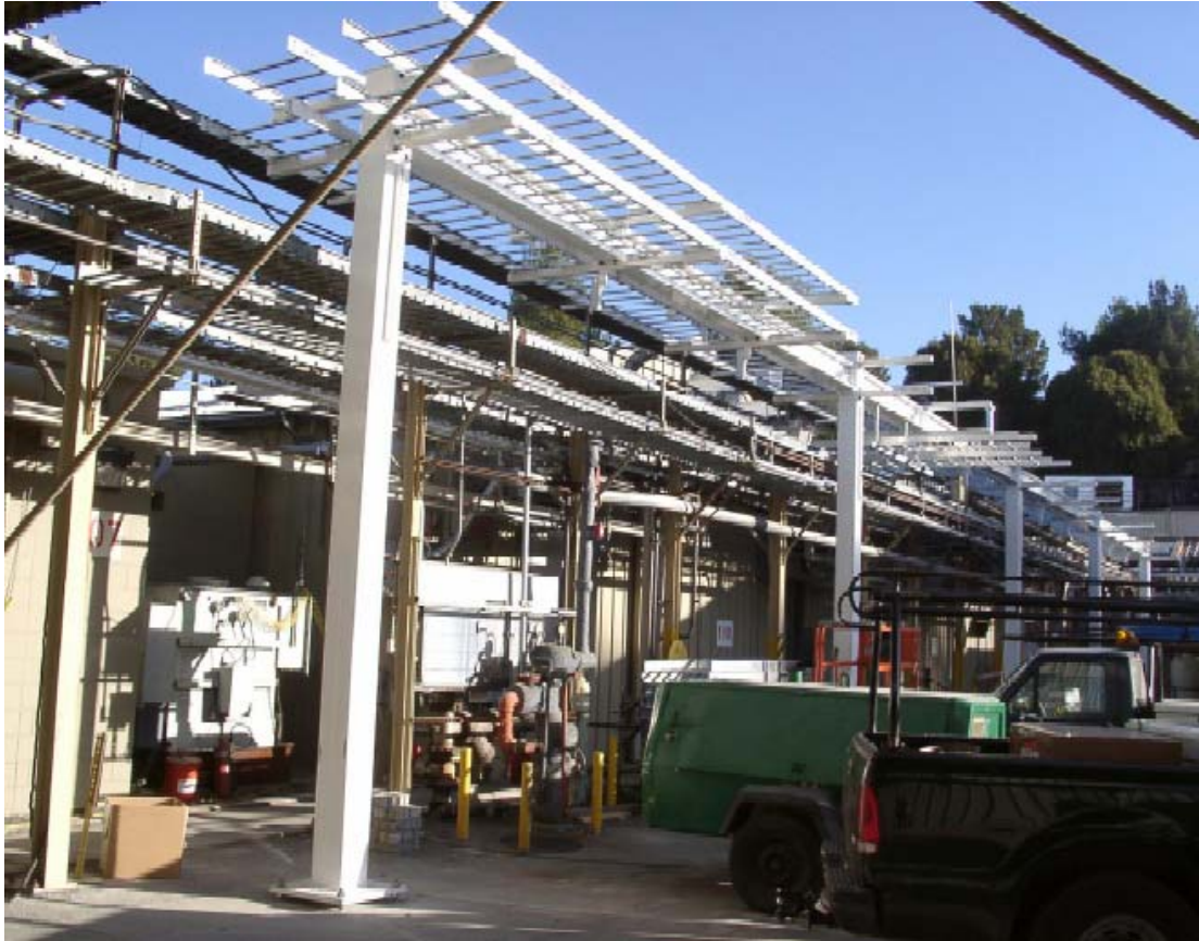
Figure 8 – New cable trays in construction
