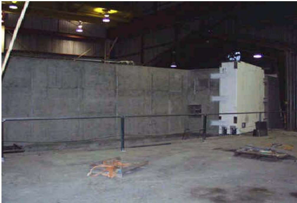
Figure 6 – Completed west straight section outer wall with future beam line port
