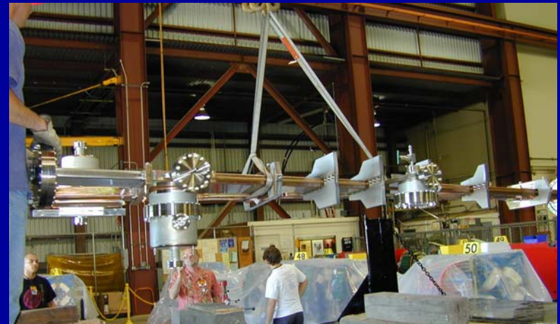
BM-1 chamber installation
