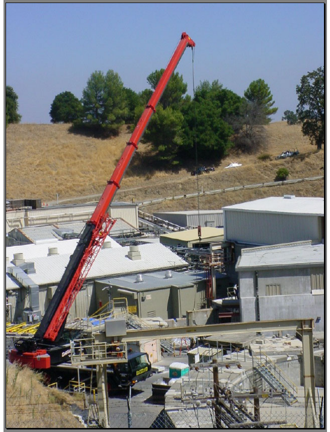
New ID & shielding blocks being installed in South Arc of SPEAR using the large 150T crane
