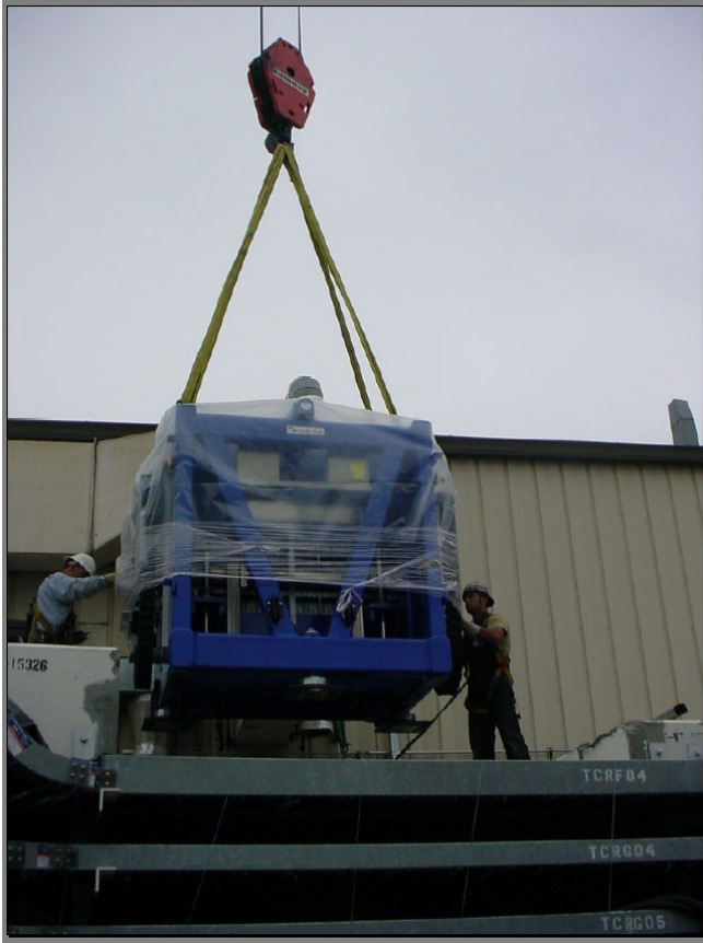
New ID & shielding blocks being installed in South Arc of SPEAR using the large 150T crane
