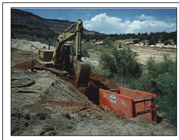
**Figure 1.** Top: schematic diagram of a permeable reactive barrier. Bottom: installation of the apatite PRB at Fry Canyon, Utah.
