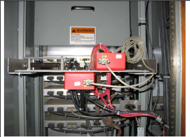
Picture 2.4 New TSP power supply installation.
