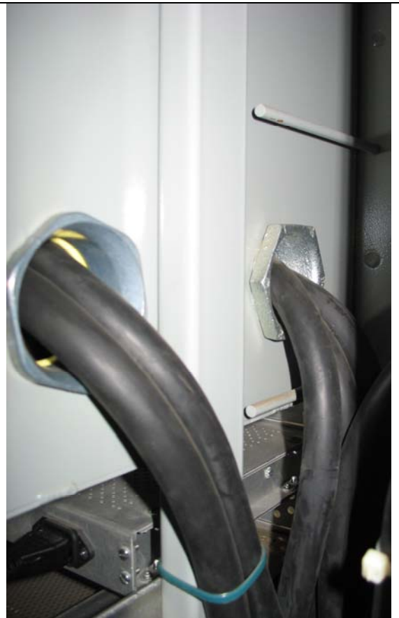
Picture 2.3b New cable penetration on AC distribution box.
